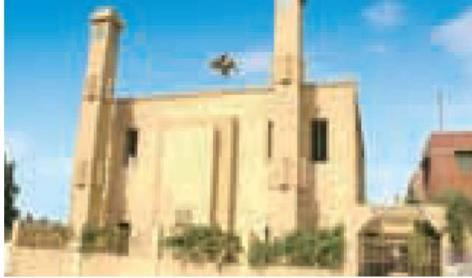
Mosque - near IIL Factory
